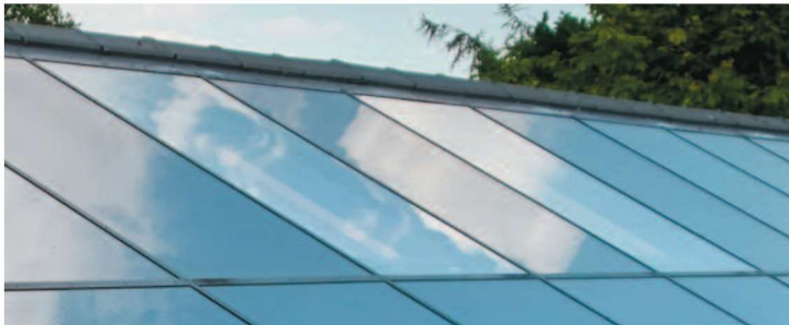
For passive houses, a popular option is to use inward-opening triple glazed roof windows, set under a clear glass unit instead of a solar panel.
